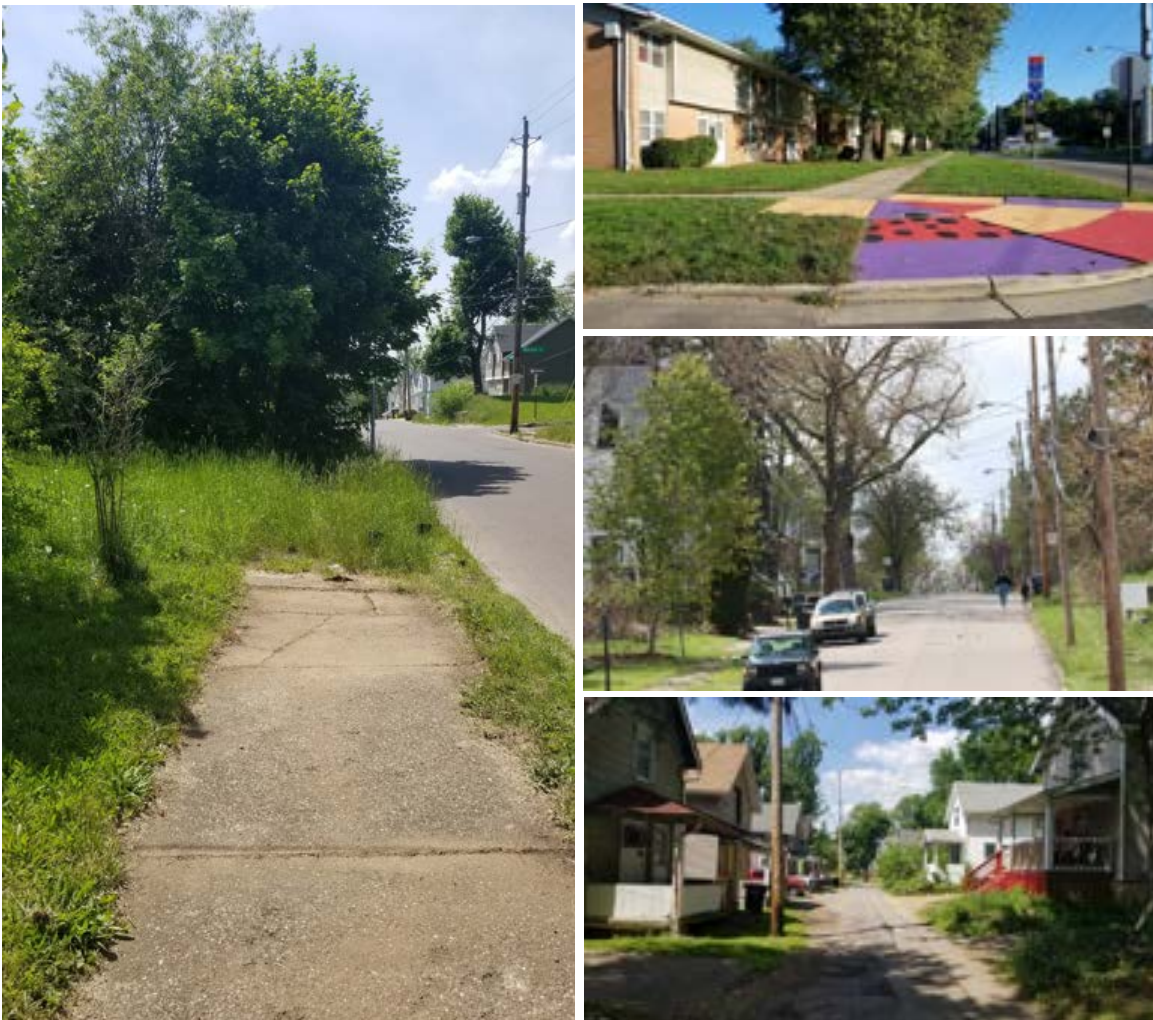
Examples of sidewalk conditions.
