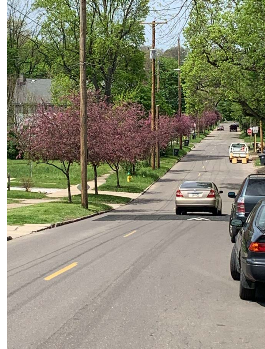
New speed tables installed on Miller Avenue
